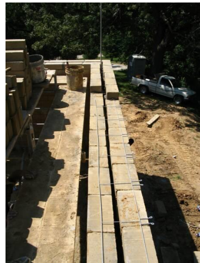
Figure 1 Double wall prior to insulation
